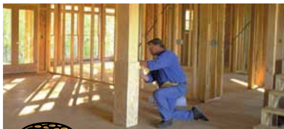
NEW HOME CONSTRUCTION
